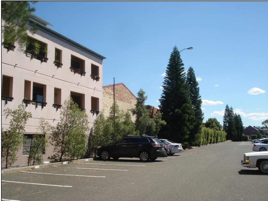
Figure 6 – Adjoins residential developments at Daphne Street
